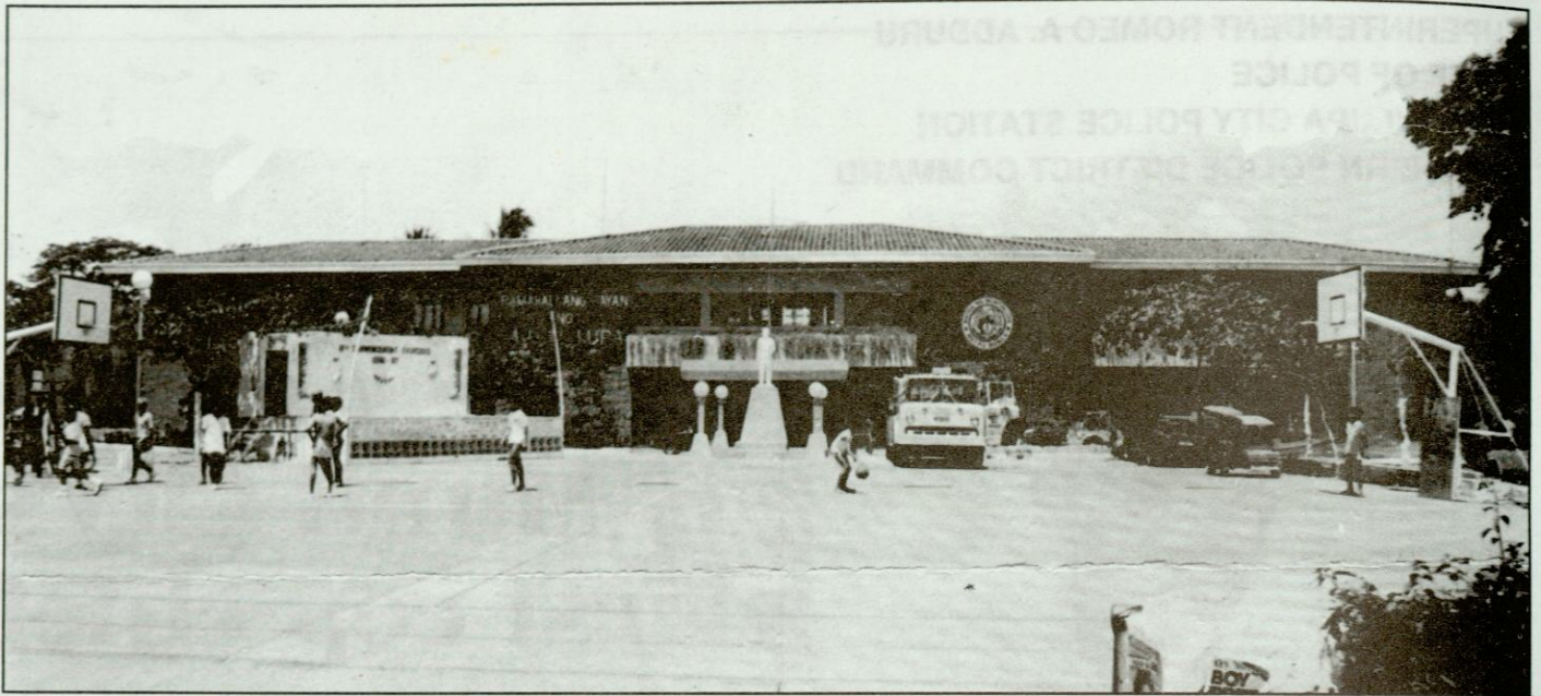
MUNTINLUPA CITY HALL. A panoramic view of the Muntinlupa City Hall along the National Road, Barangay Putatan, Muntinlupa.
